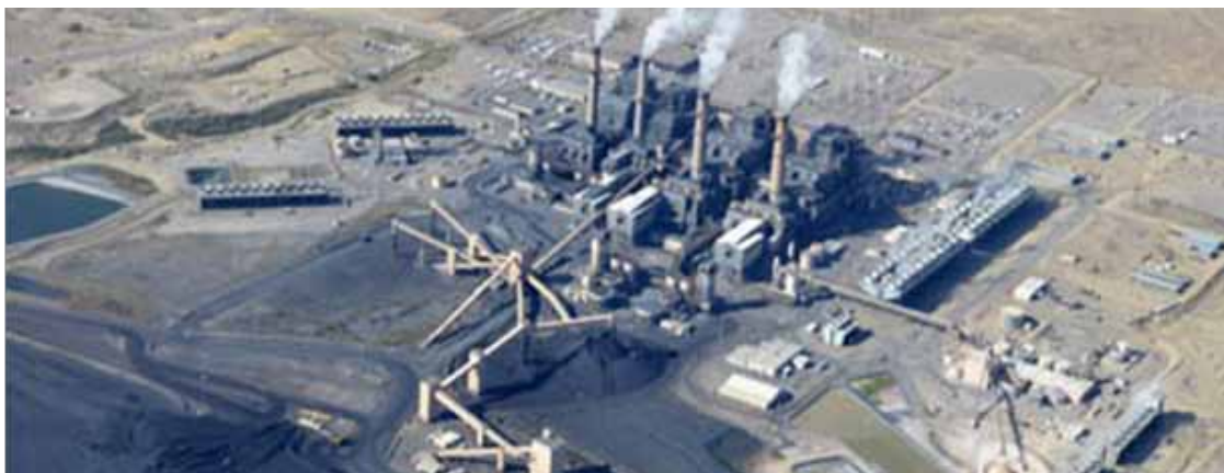
The San Juan Generating Plant, New Mexico USA, example of Mine Mouth Power Plant
