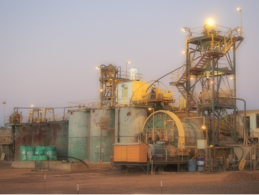
Refurbished and operational processing plant
