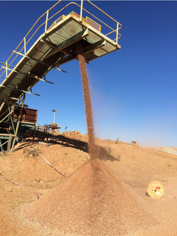
Crushing circuit refurbished and operational
