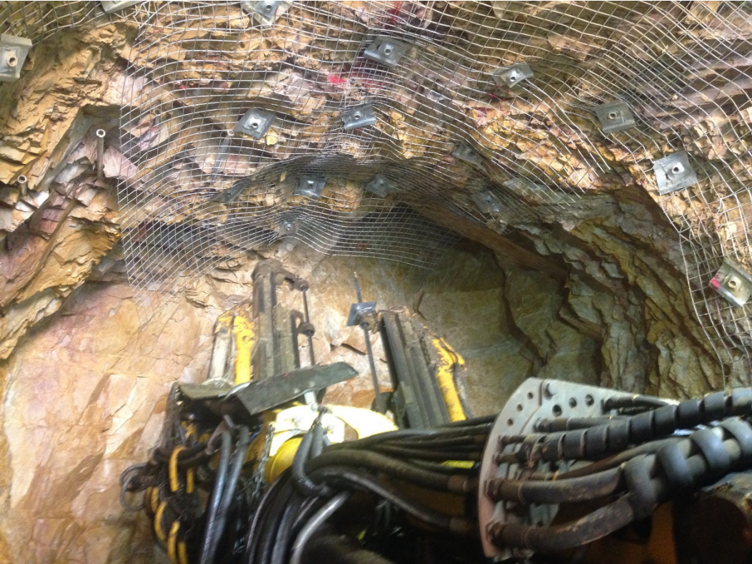
Meshing decline backs at Nicolson’s underground operation
