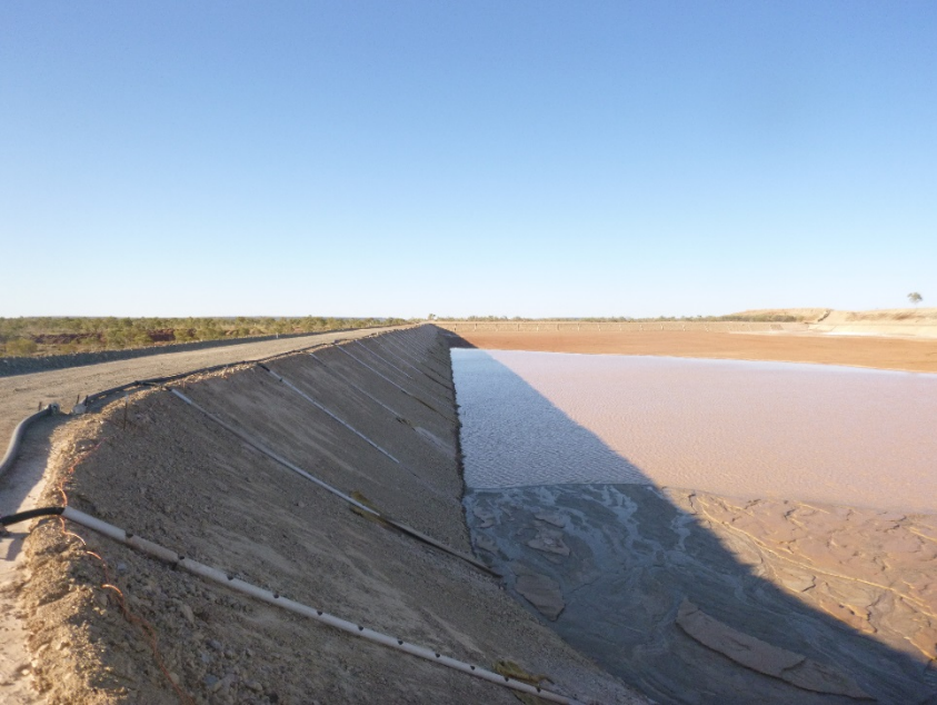
Refurbished tailings dam
