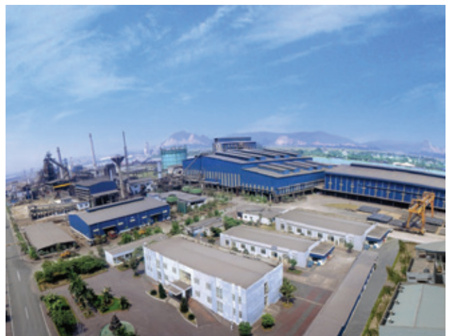
HPG Hoa Phat Steel Integrated Complex in Hai Duong
