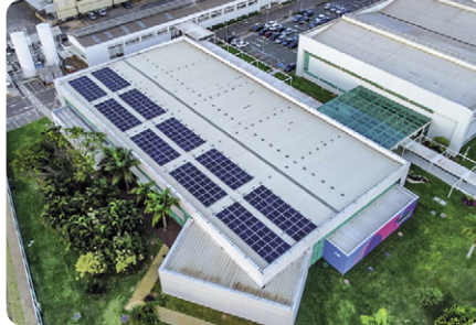
Solar photovoltaic array in São Carlos
