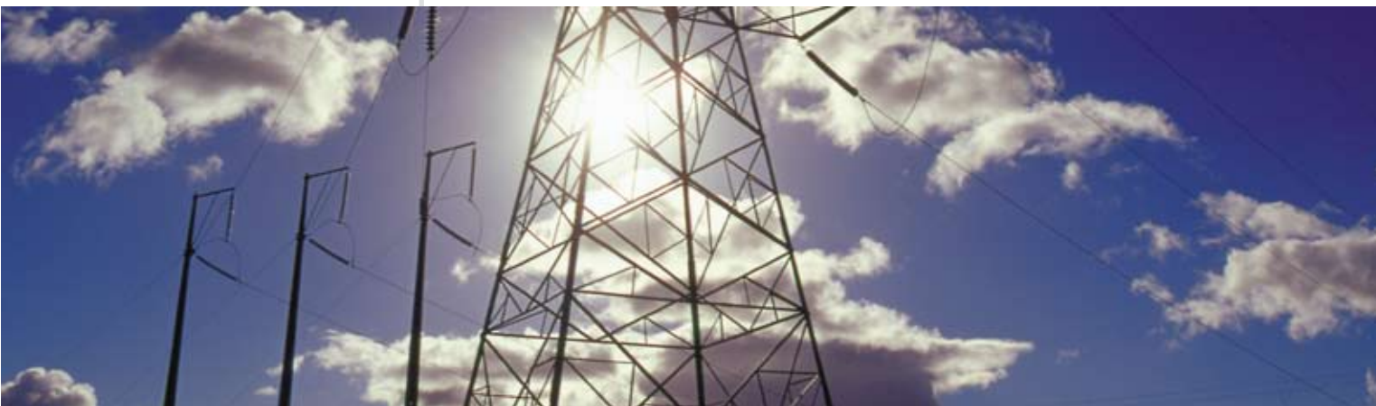
Chesf Transmission Lines (Chesf Files)
