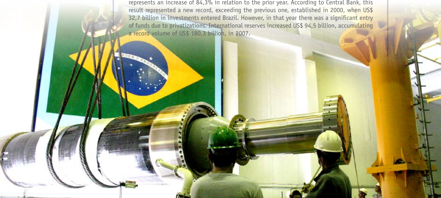
Eletronuclear – Generator Rotor of the Nuclear Plant Angra 2 (Eletronuclear Files)
