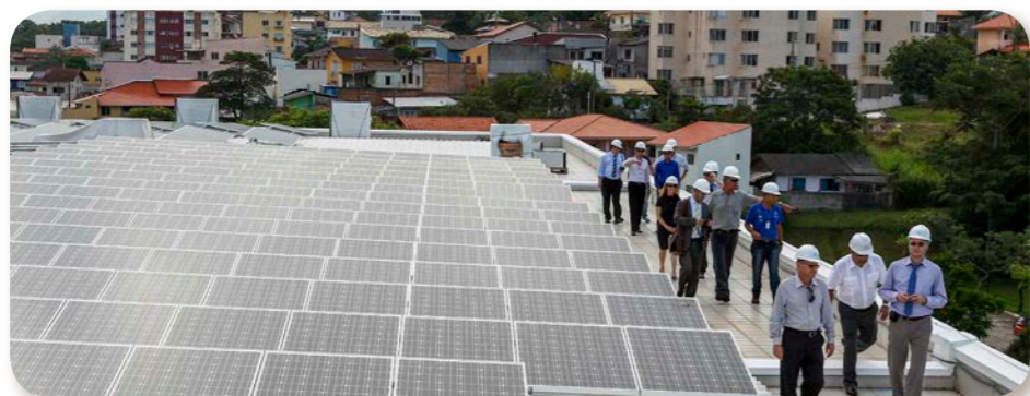
Megawatt Solar Plant, located in the headquarters of Eletrobras Eletrosul in Florianópolis (SC)
