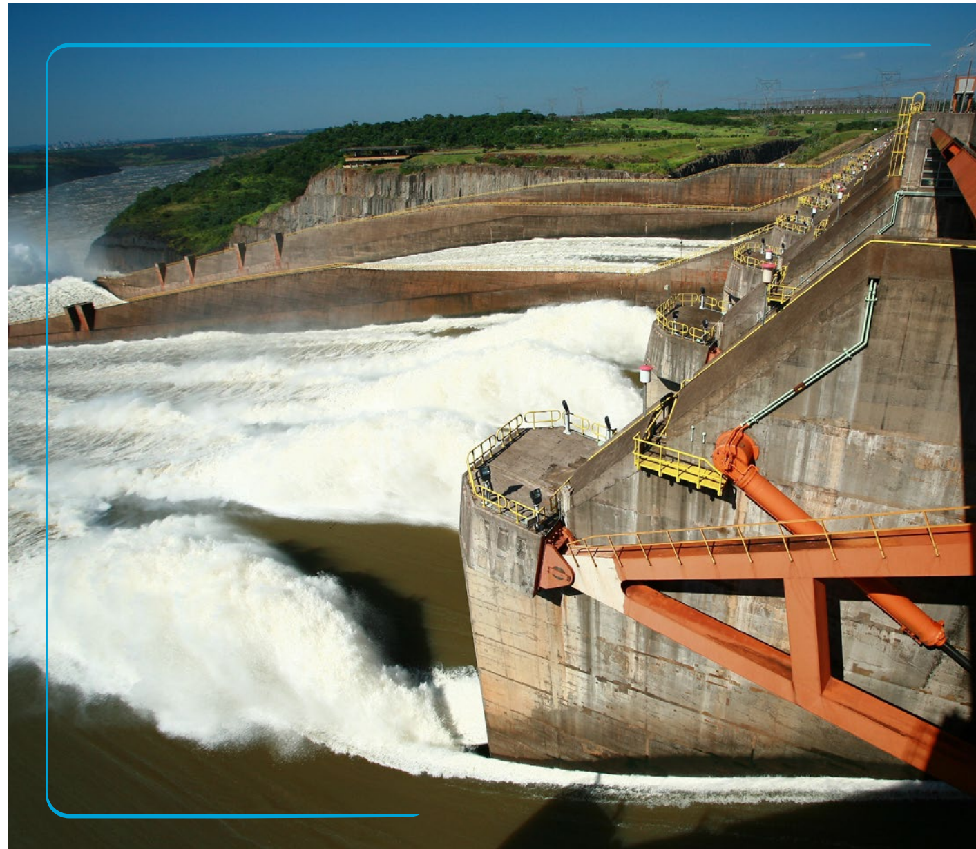
Panorama of the spillway springboard of the Itaipu hydroelectric plant. Itaipu Binacional / Caio Coronel collection.
