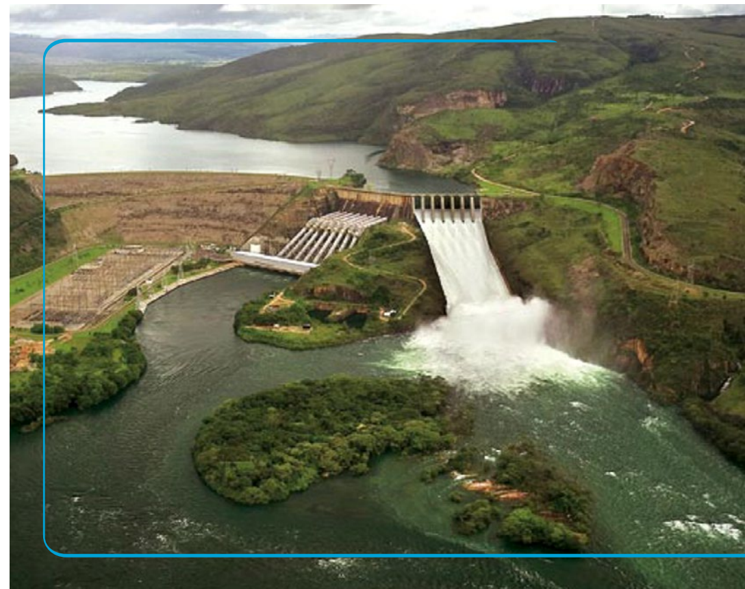
Furnas hydroelectric plant. Eletrobras Furnas Collection.
