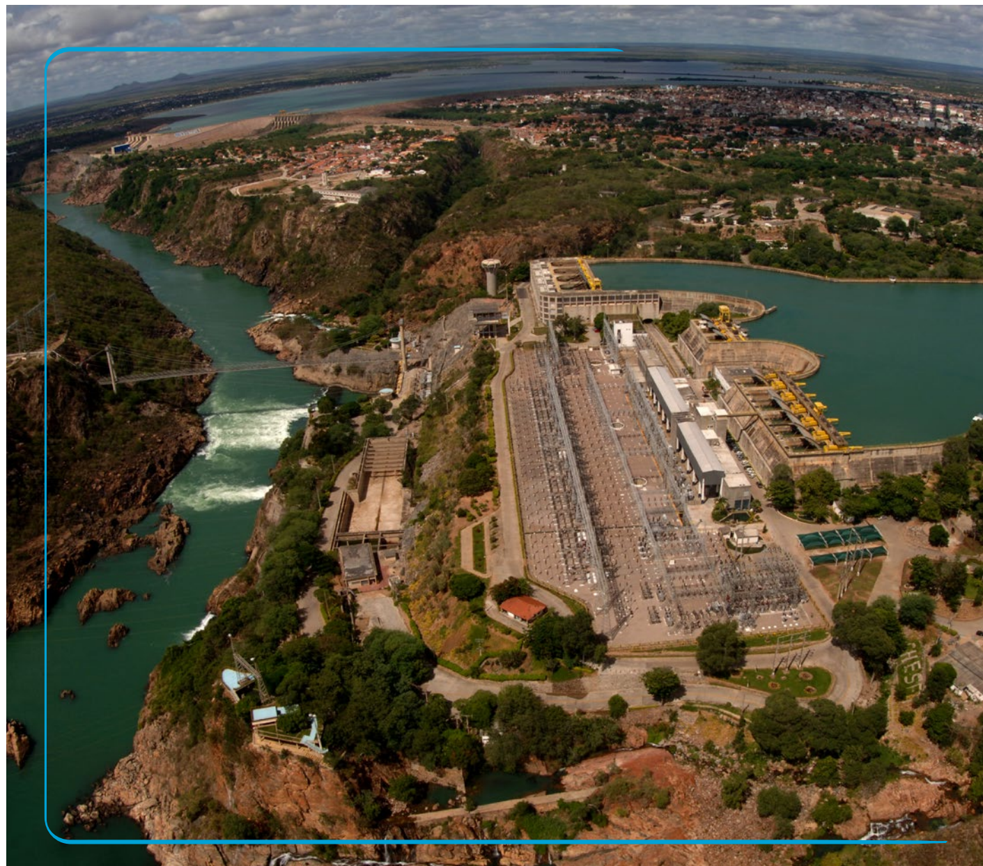
Hydroelectric complex Paulo Afonso. Eletrobras Chesf/ Severino Silva Collection.
