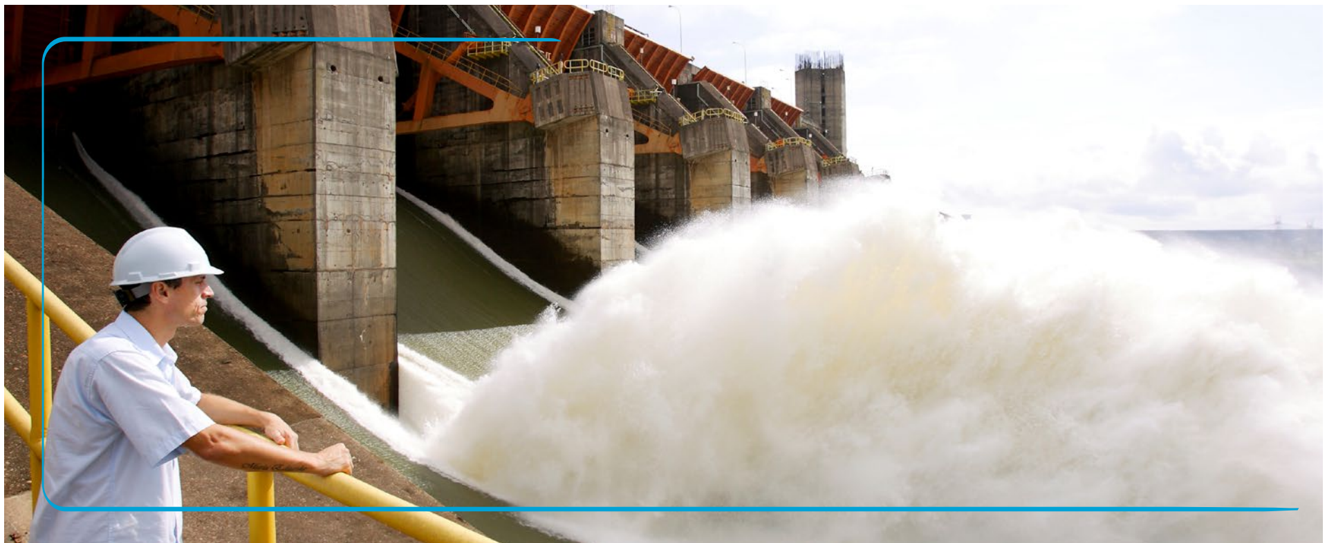
Spillway of the Itaipu Hydroelectric Plant. Itaipu Binacional / Caio Coronel collection.
