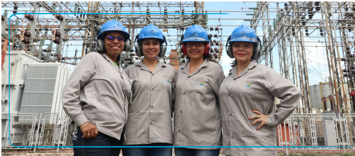
Substation workers. Amazonas GT Collection.
