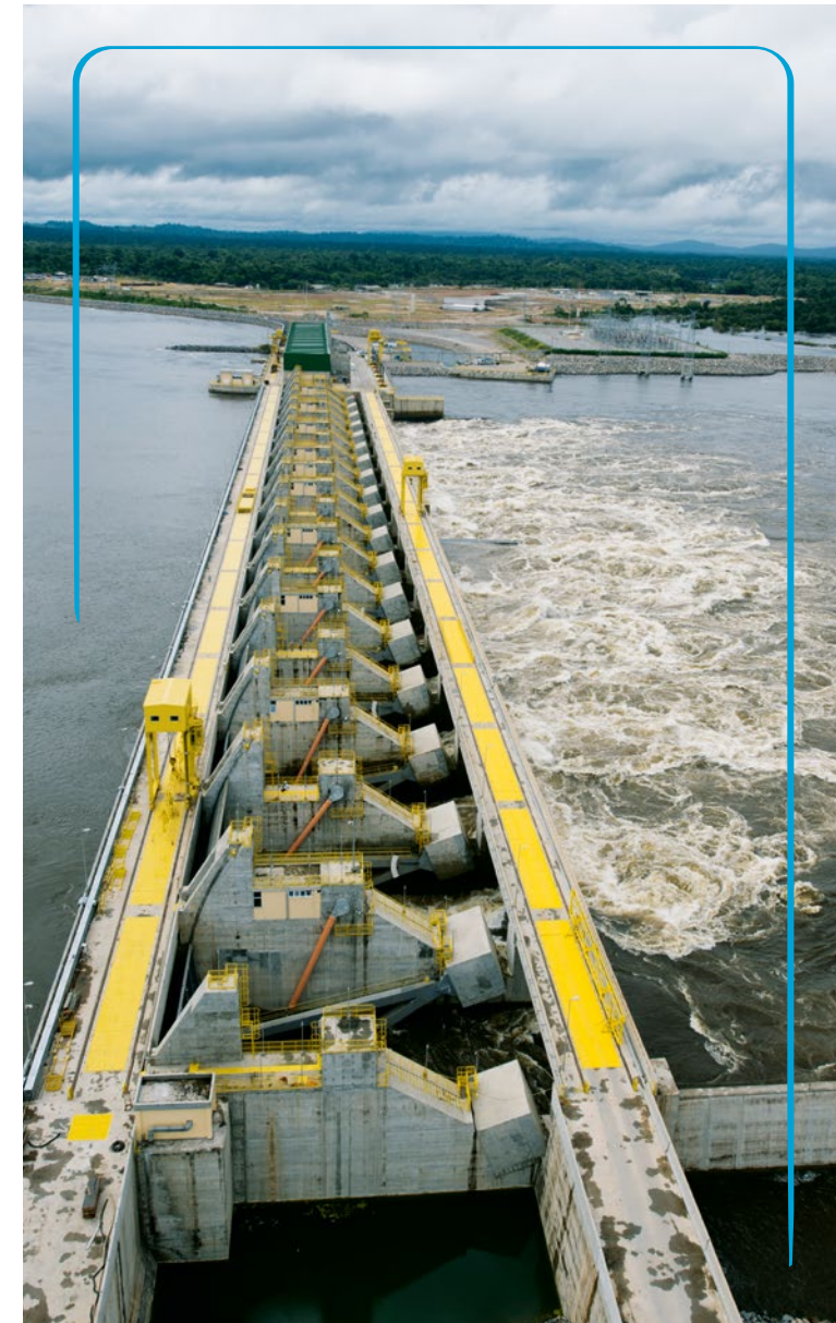
Belo Monte hydroelectric plant. Norte Energia Collection / Betto Silva.
