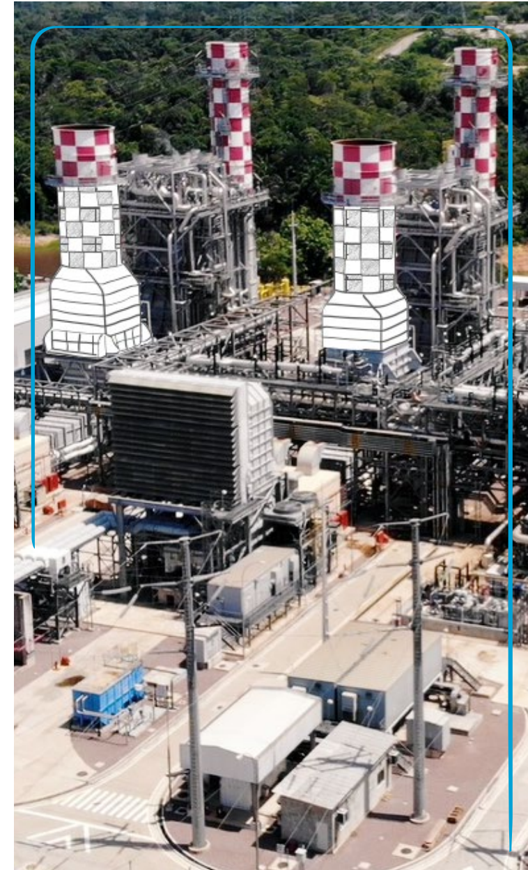
Mauá thermal power plant 3. Eletrobras Amazonas GT Collection.
