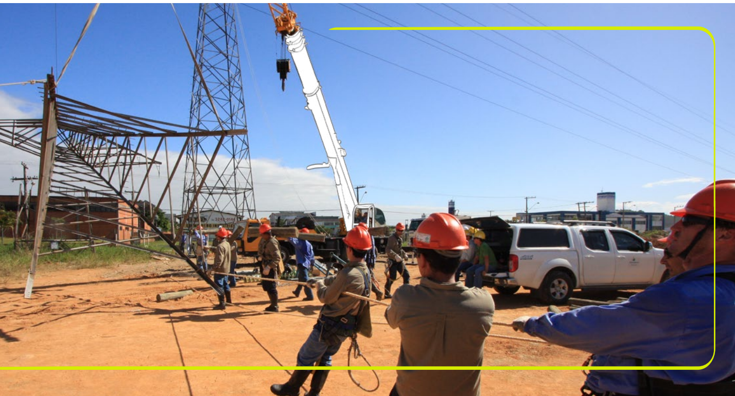
Exchange of transmission towers. Eletrobras CGT Eletrosul Collection.
