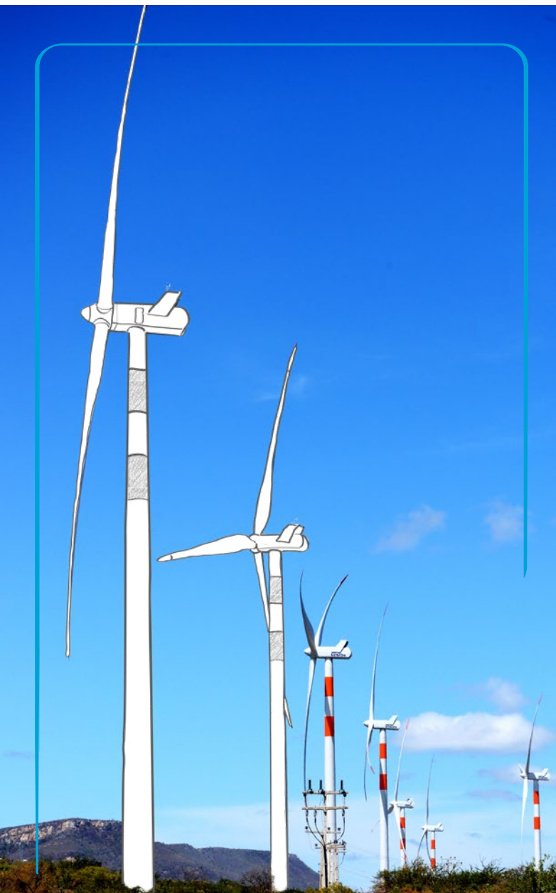
Sento Sé Wind Complex. Eletrobras Chesf / Severino Silva Collection.
