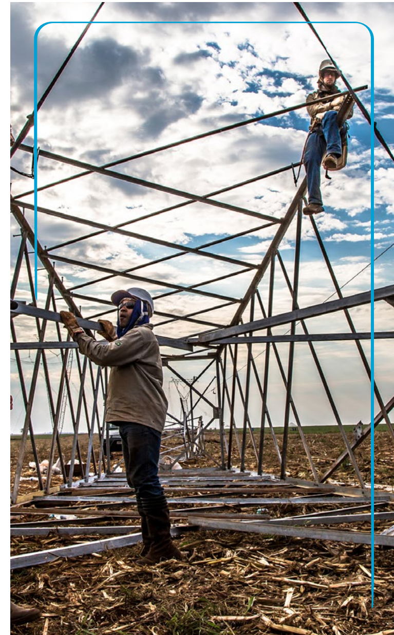
Transmission tower maintenance. Eletrobras Furnas Collection / Daniela Monteiro.
