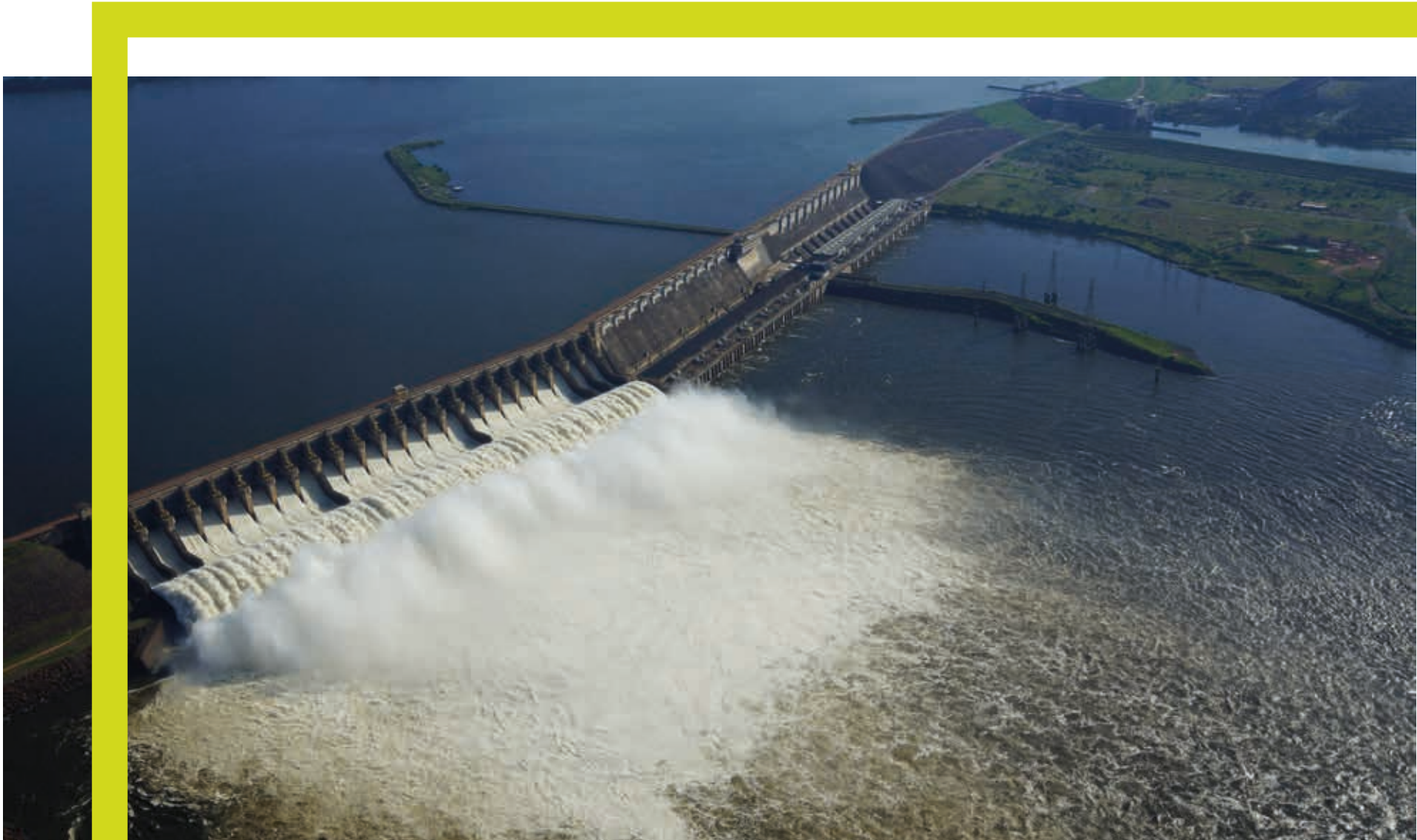
The Tucuruí Dam. Photo: Rony Ramos
