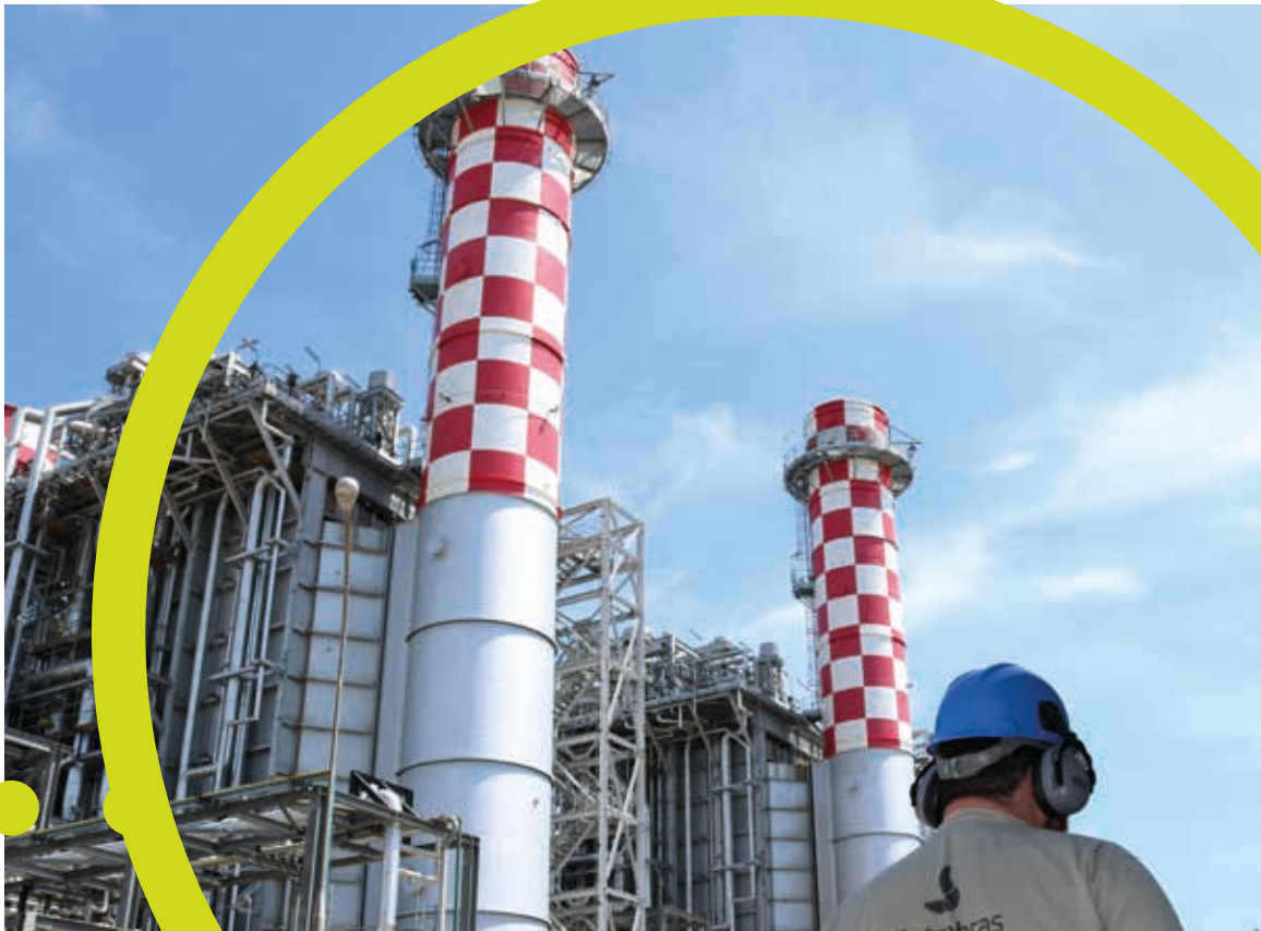
The Mauá thermal power plant. Amazonas GT Archives.
