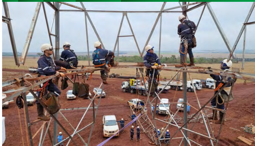
Linemen working on an Eletrobras Furnas transmission tower. Photo: Alexandro Rodrigues.
