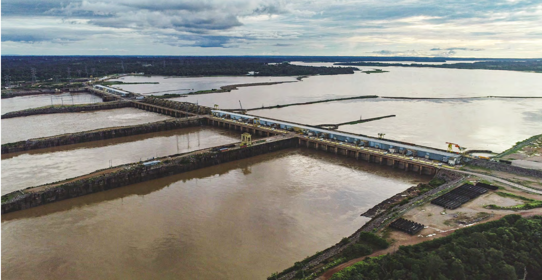
Overhead view of Eletrobras Furnas' Santo Antônio hydroelectric dam. Photo: Eletrobras Furnas Archives.
