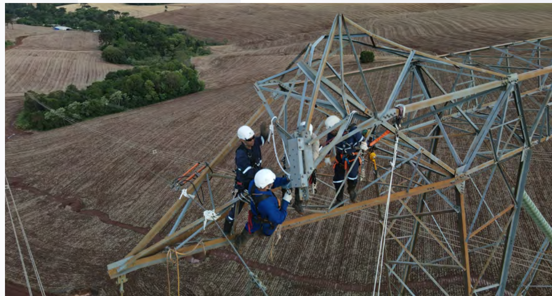
An Eletrobras CGT Furnas lineman crew. Photo: Alexandre Rodrigues
