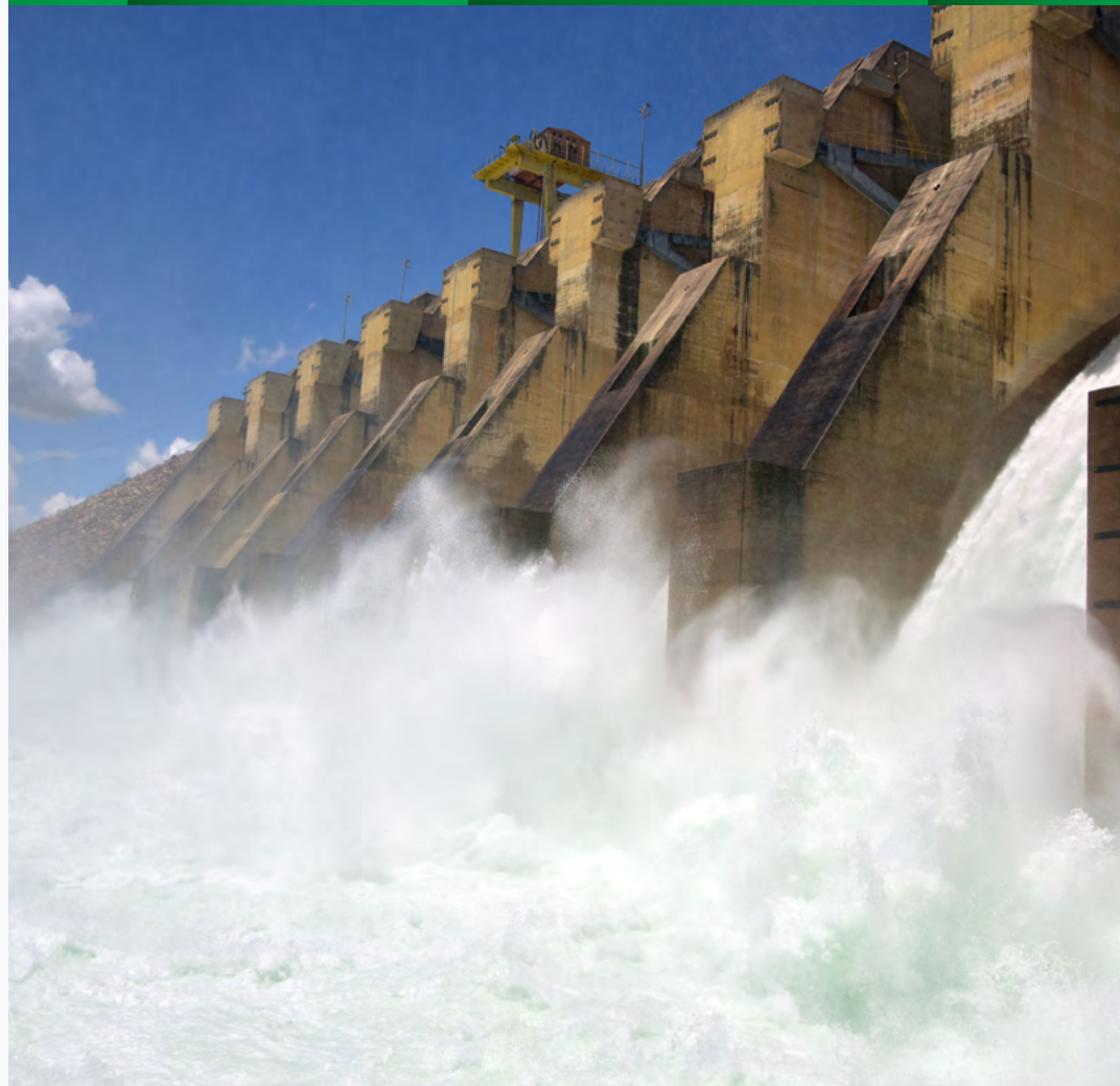
The spillway of the Eletrobras Chesf's Luiz Gonzaga Dam. Photo: Andre Schuler.
