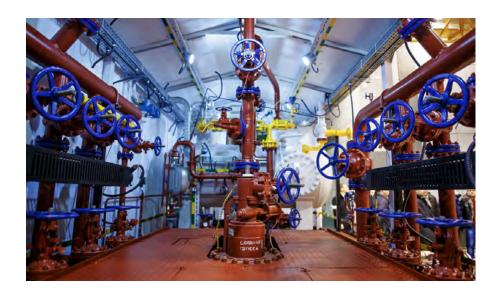
of pressure maintenance operations and is equipped with five CNS type centrifugal multistage pumps with 240 m3/h capacity and 1422m pressure head. The station consists of highly prefabricated process and electrical skid modules for short transportation and installation time. An automatic control system ensures operation of the equipment without continuous presence of personnel.
