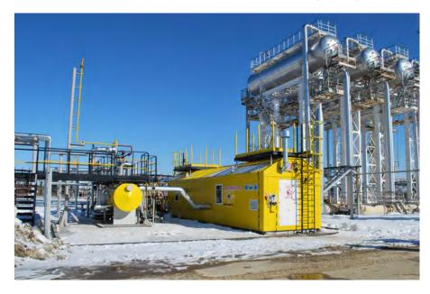
Compressor station with liquid-ring compressor for Rosneft
