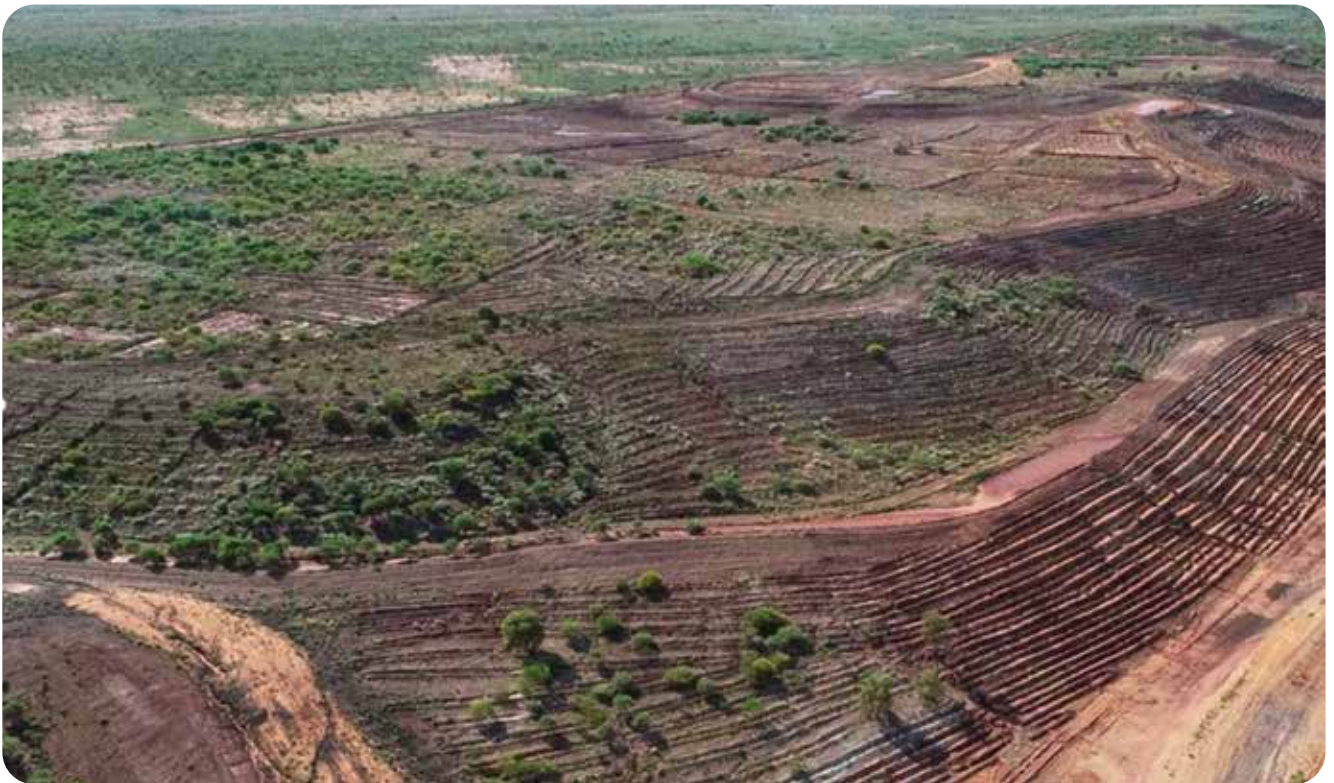
Chugga WRD (looking South)
