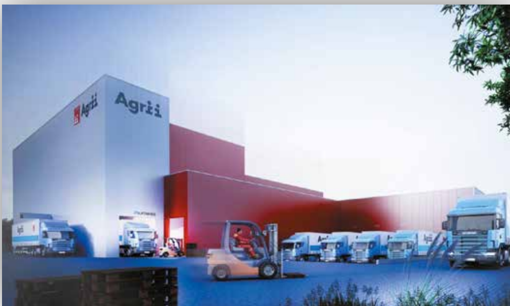
Design concept of Agrii's new state-of-the-art specialised seed processing and input formulation facility in Aleksandrów, Poland.
