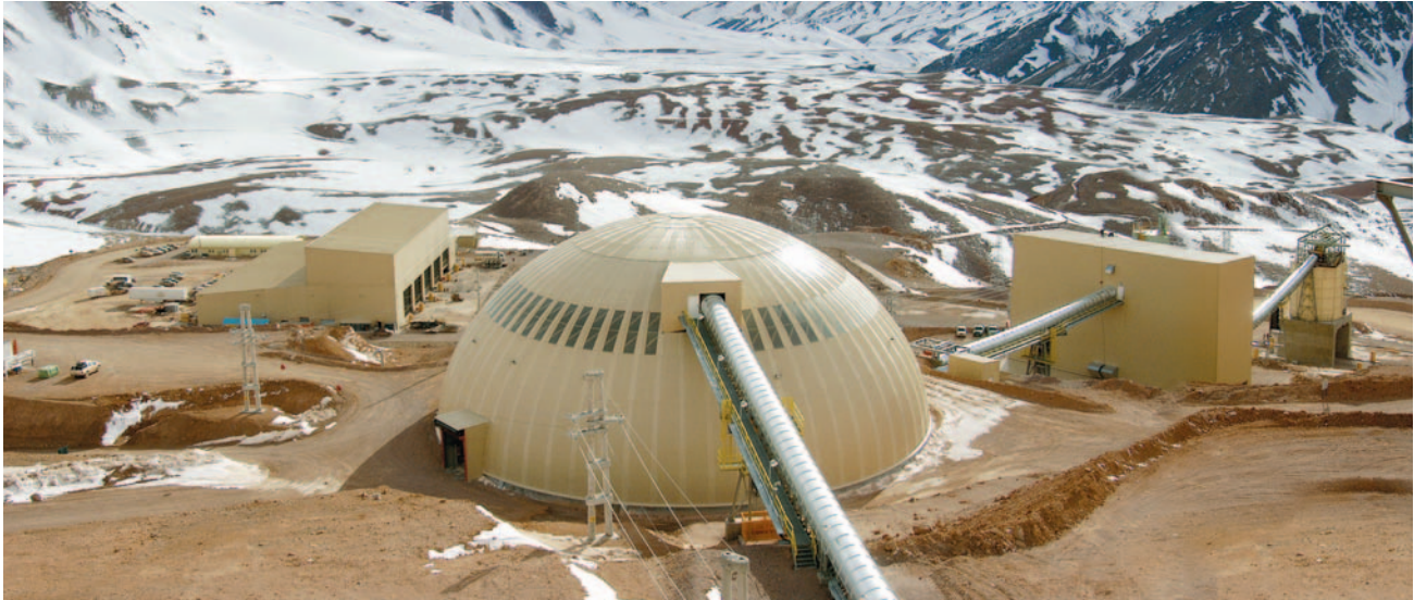
Infrastructure at Veladero, Argentina (left to right): the truck shop, the covered ore stockpile, the secondary crusher and the loadout bin, where trucks collect crushed ore to haul to the valley-fill leach facility. 2006 will be the mine's first full year of production.
