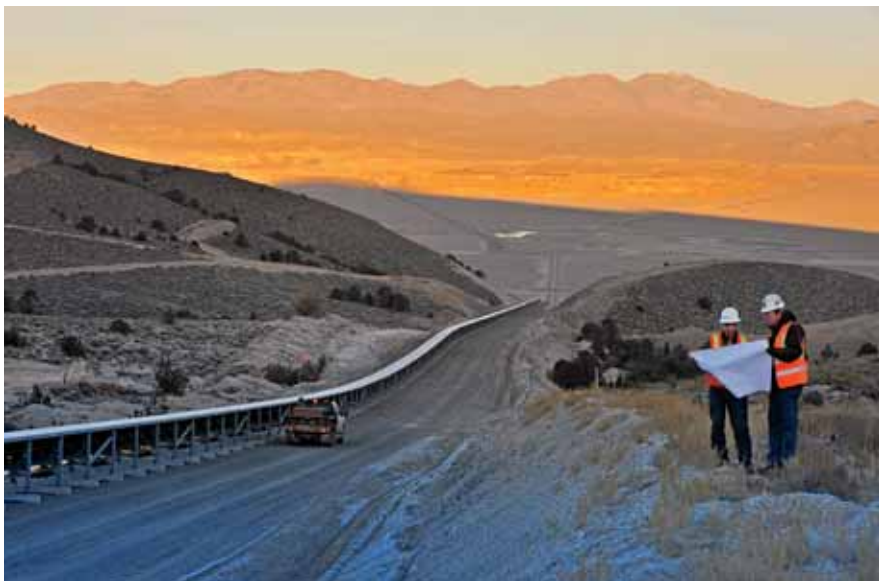
The 15 kilometer ore conveyor transports crushed material from the Cortez Hills deposit across Crescent Valley to the processing facilities at the existing Cortez mine.
