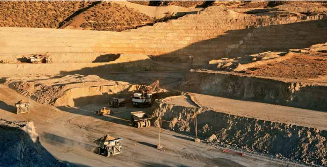
Cortez Hills is expected to materially benefit Barrick’s overall production and cost profile. The existing process infrastructure blends ore from the Pipeline deposit with ore from Cortez Hills.
