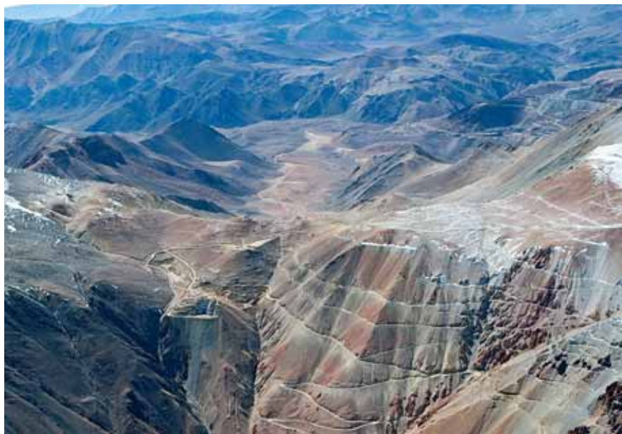
A platform is already in place and the portal for the ore conveyor tunnel, shown in the foreground of this photo, has been completed. The tunnel will be used to transport the ore from Chile into Argentina where the process facilities will rest in the valley beyond. Close proximity to Veladero is shown with the Filo Federico pit in the upper right.
