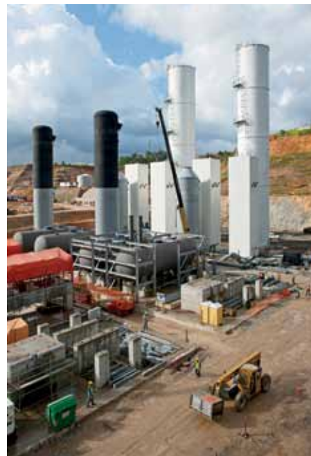
High purity oxygen from the plant will be injected into the Pueblo Viejo autoclaves to release the gold.
