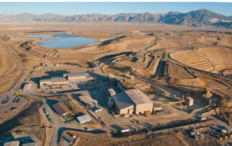
The Cortez mine in Nevada exceeded expectations for the third straight year. The processing facilities are shown in the foreground.
