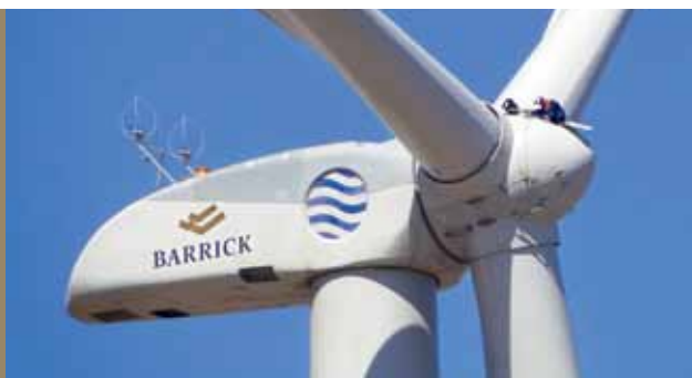
Barrick's $50 million Punta Colorado wind farm in Chile.
