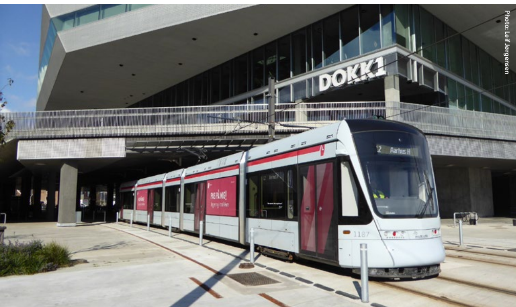
Ricardo Certification was the Independent Safety Assessor for the recently opened Phase 2 of the light rail project connecting the cities of Aarhus and Odder in Denmark
