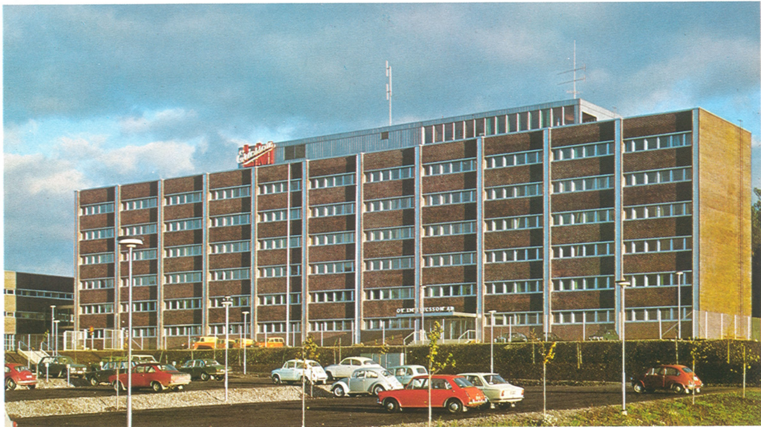
Ericsson's Finnish subsidiary, Oy L M Ericsson Ab, occupied its new factory and office facilities at Jorvas, near Helsinki, during 1971. The plant is designed for 800 factory employees and the office section for 350.
