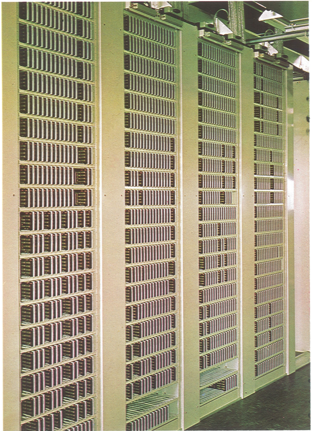
Ericsson's first computer-controlled (AKE 13) telephone exchange for wholly automatic switching of long distance and international traffic was inaugurated in Rotterdam during the year. The exchange can handle more than half a million calls in a 24-hour period. Picture shows racks mounted with circuit cards containing miniature components.
