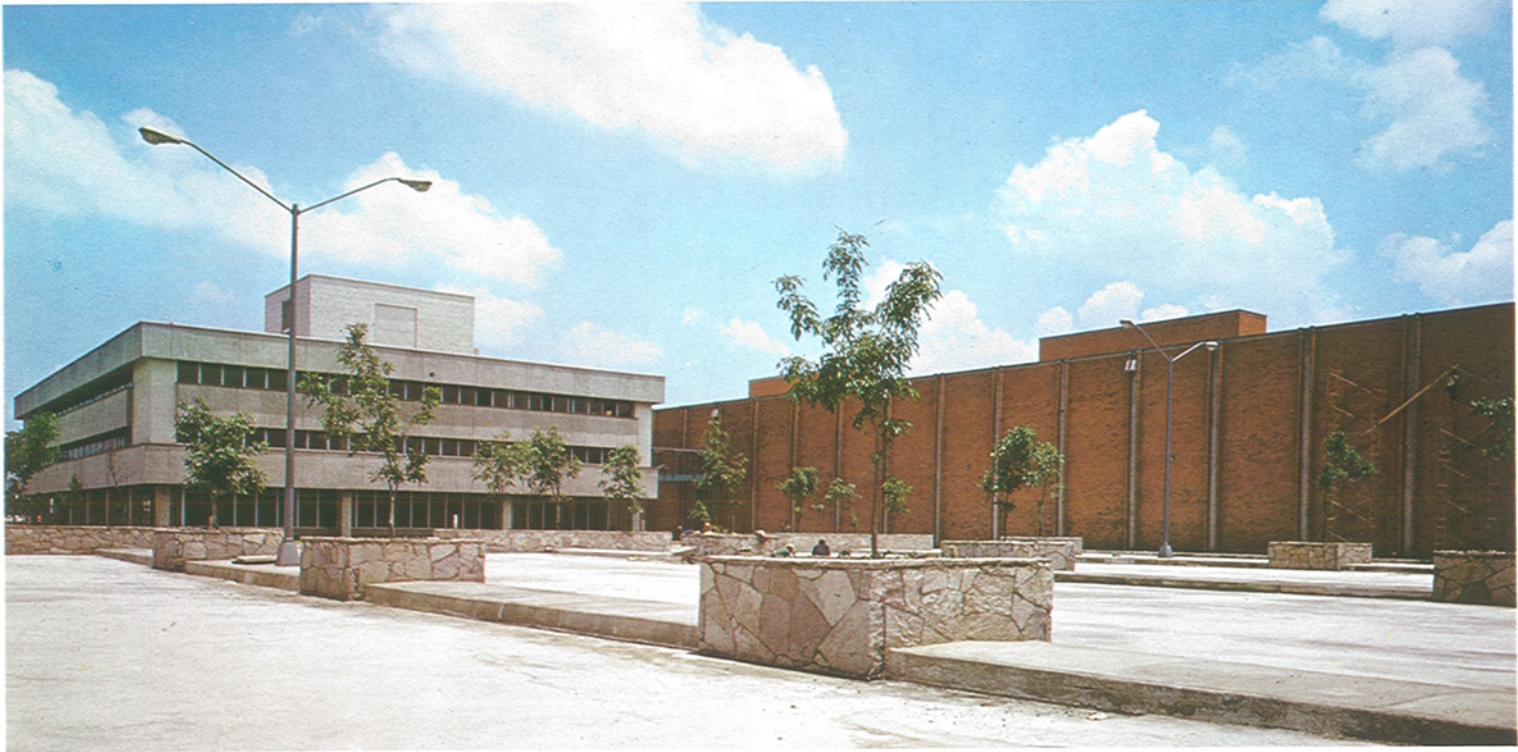
A new factory and office complex for Teleindustria S.A., a Mexican subsidiary, was completed during the year. The complex, which includes a training center, is located at Tlalnepantla, a suburb of Mexico City. The factory unit covers 160,000 sq.ft.
