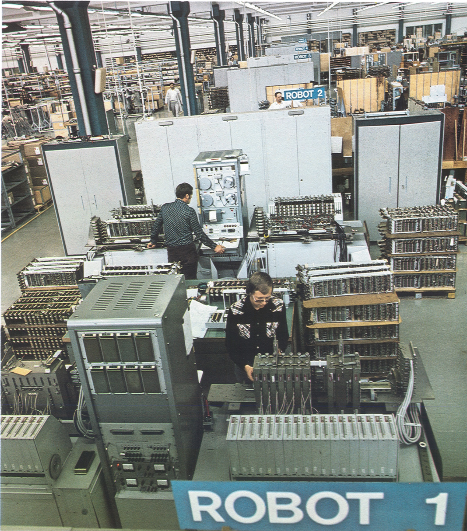
Robot test equipment is used to check relay sets in Parent Company plant in Visby.
