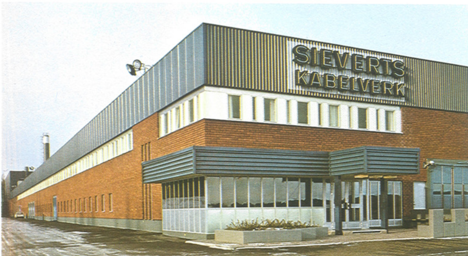
New cable plant completed recently by Sieverts Kabelverk AB at Falun, Sweden, for the production of underground plastic cable.
