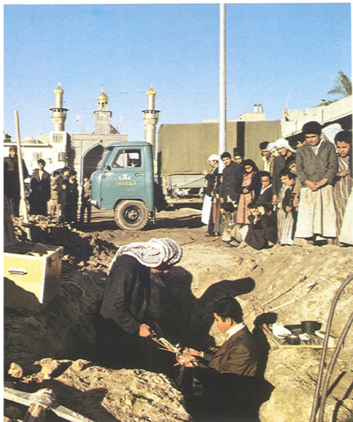
Jointing of telecommunications cable at Kerbala, Iraq.
