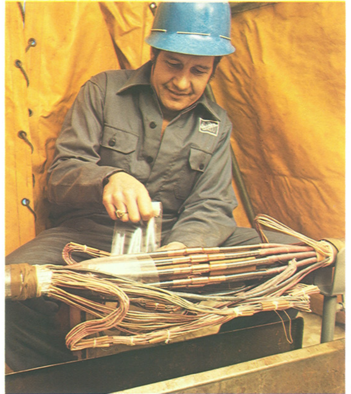
Extension of a telephone network: cable being spliced under field conditions.
