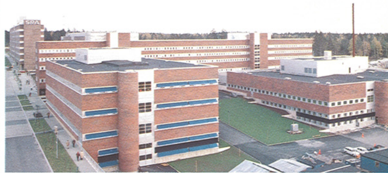
Rifa's new plant in Kista, north of Stockholm.
