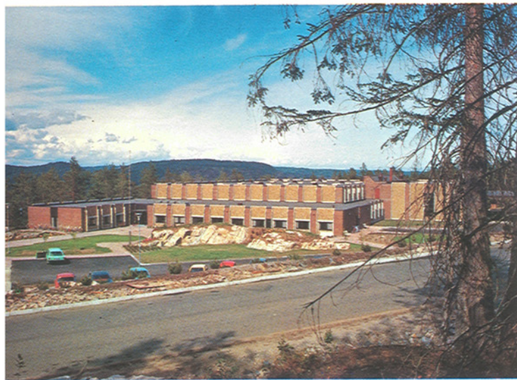
Elektrisk Bureau's new factory in Risör, Norway.
