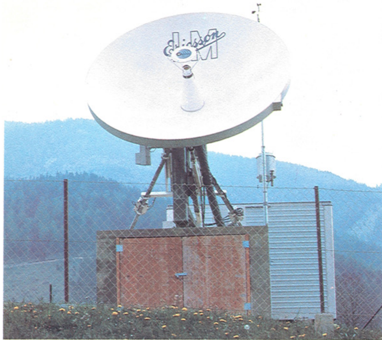
Ground station for the European OTS (Orbital Test Satellite) communications system.
