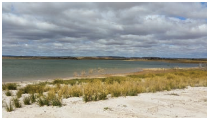
Figure 3: Retention Dam at Leigh Creek.
