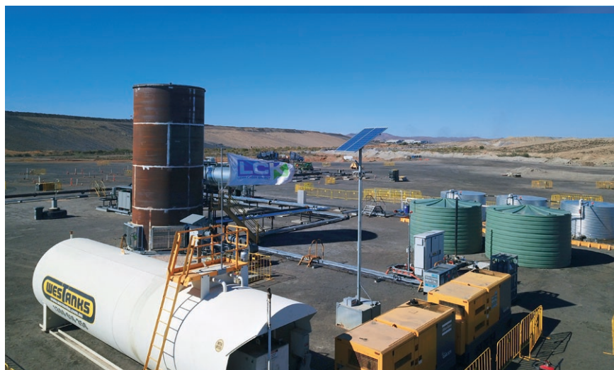
Construction site for the demonstration plant at Leigh Creek.
