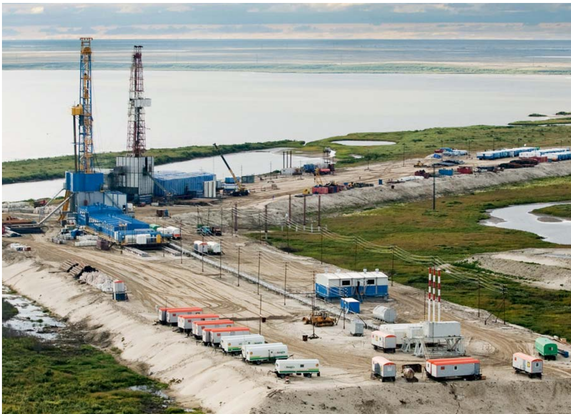
PRODUCTION DRILLING AT THE YURKHAROVSKOYE FIELD
