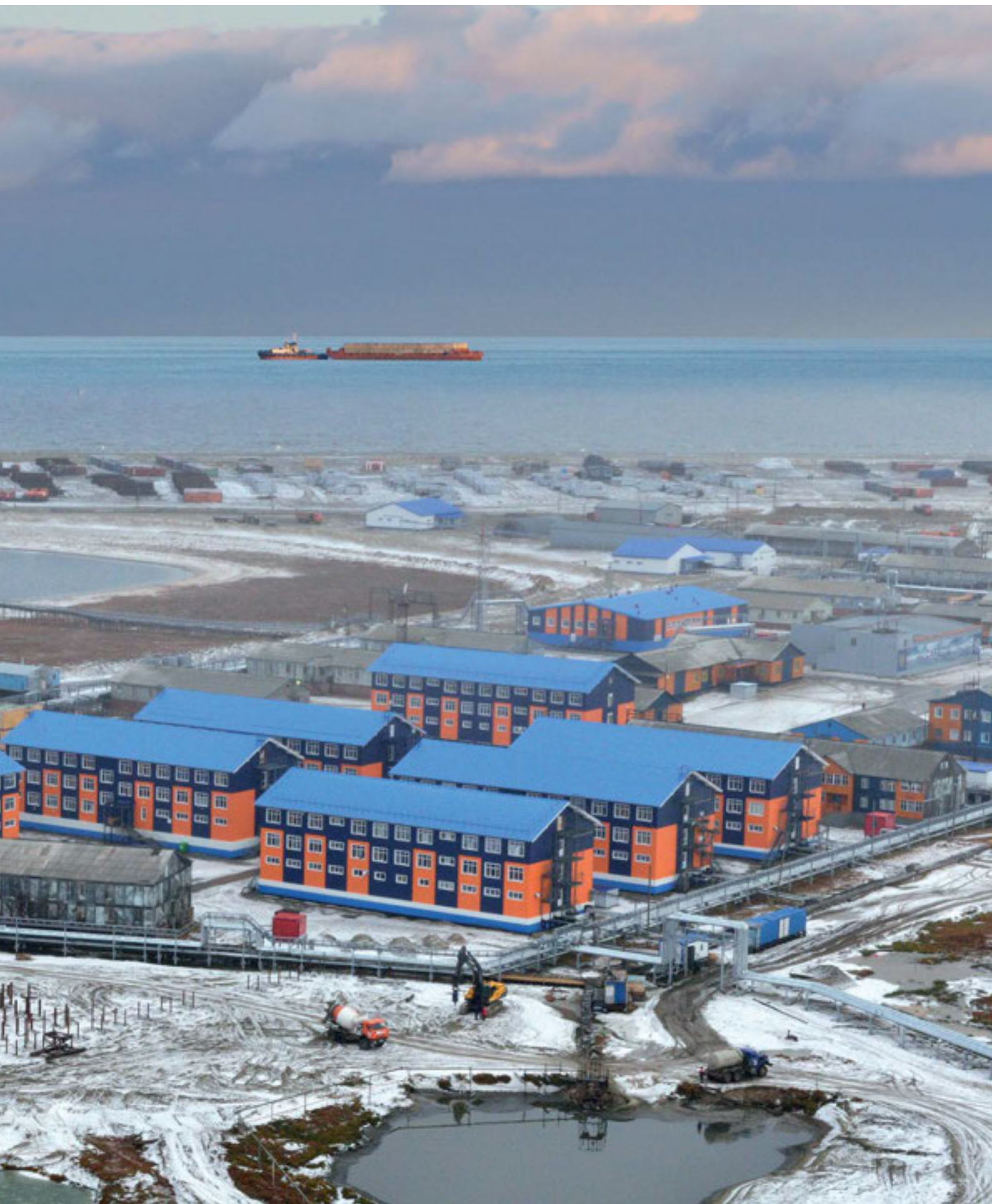
Yamal LNG, construction camp and material storage yard. September 2013
