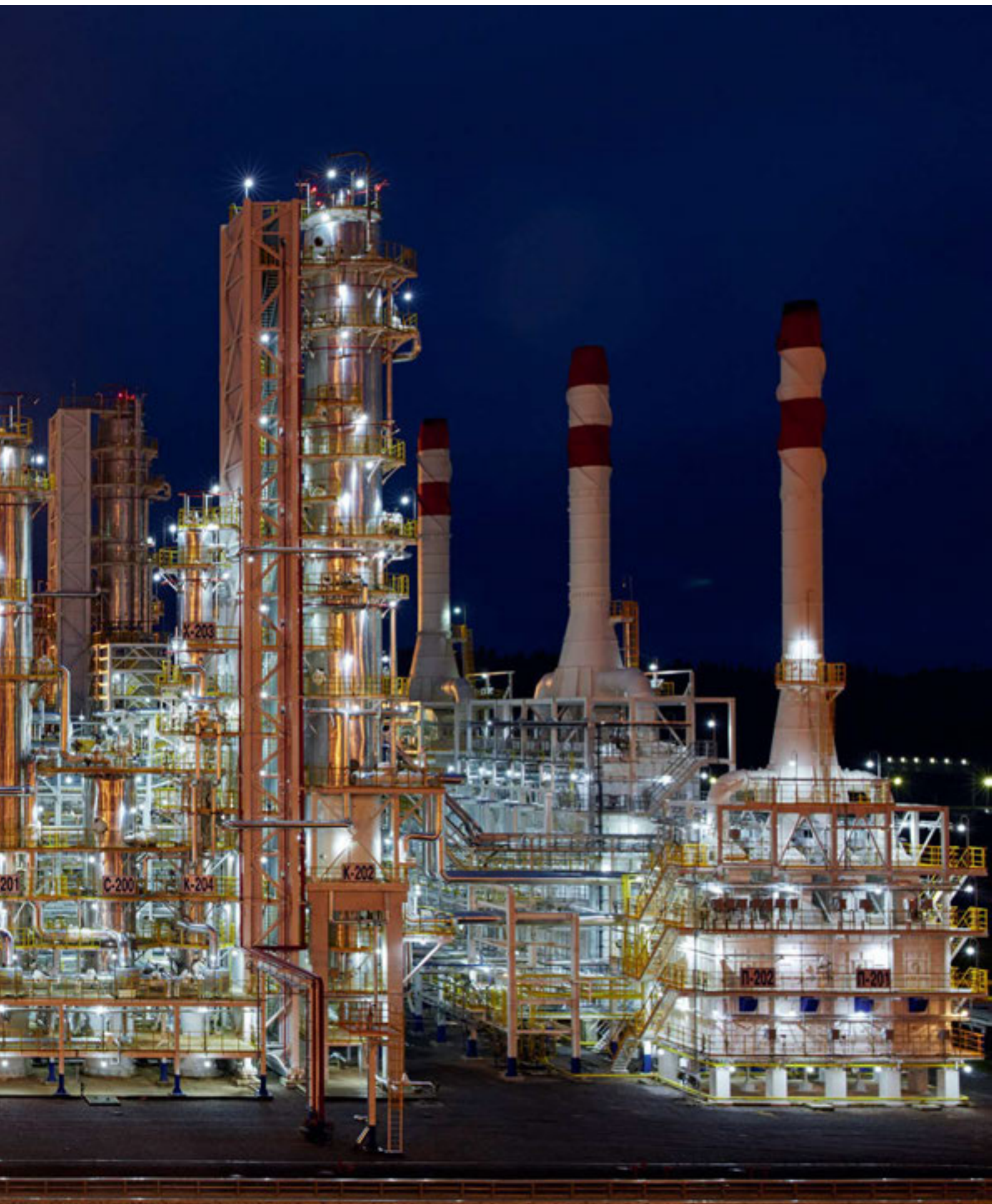
Ust-Luga Complex, stable gas condensate fractionation unit. November 2013
