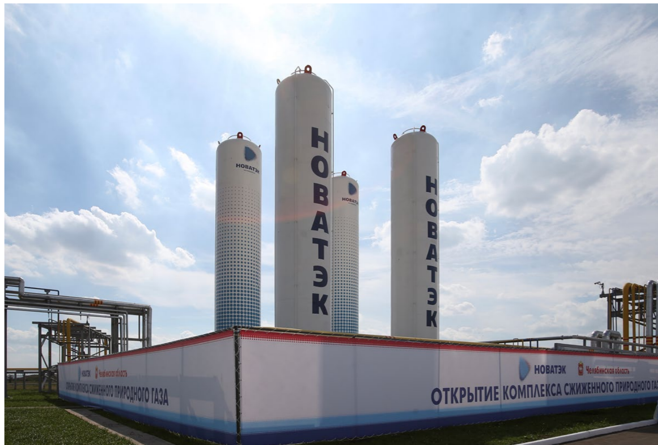
In 2020, our first small-scale LNG plant was launched in the Chelyabinsk Region (Magnitogorsk).
