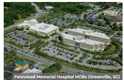
Patewood Memorial Hospital MOBs (Greenville, SC)
