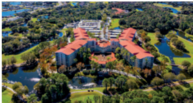
FREEDOM PLAZA SUN CITY CENTER, SUN CITY CENTER, FL
