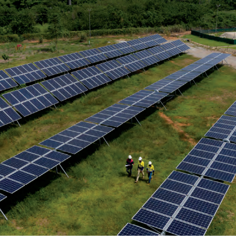
Photos (left): Employees walk through Newmont's solar panel farm in Ghana.
