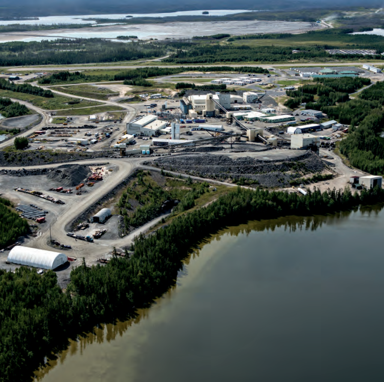
Photos (top to bottom): Aerial view of Musselwhite mine; employees in Ghana engage in enhanced COVID-19 health measures; the processing plant at Tanamai mine.
