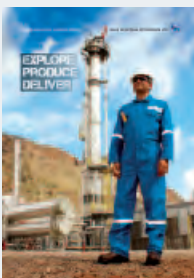
Front cover Shaikan production facility ("PF-1")
