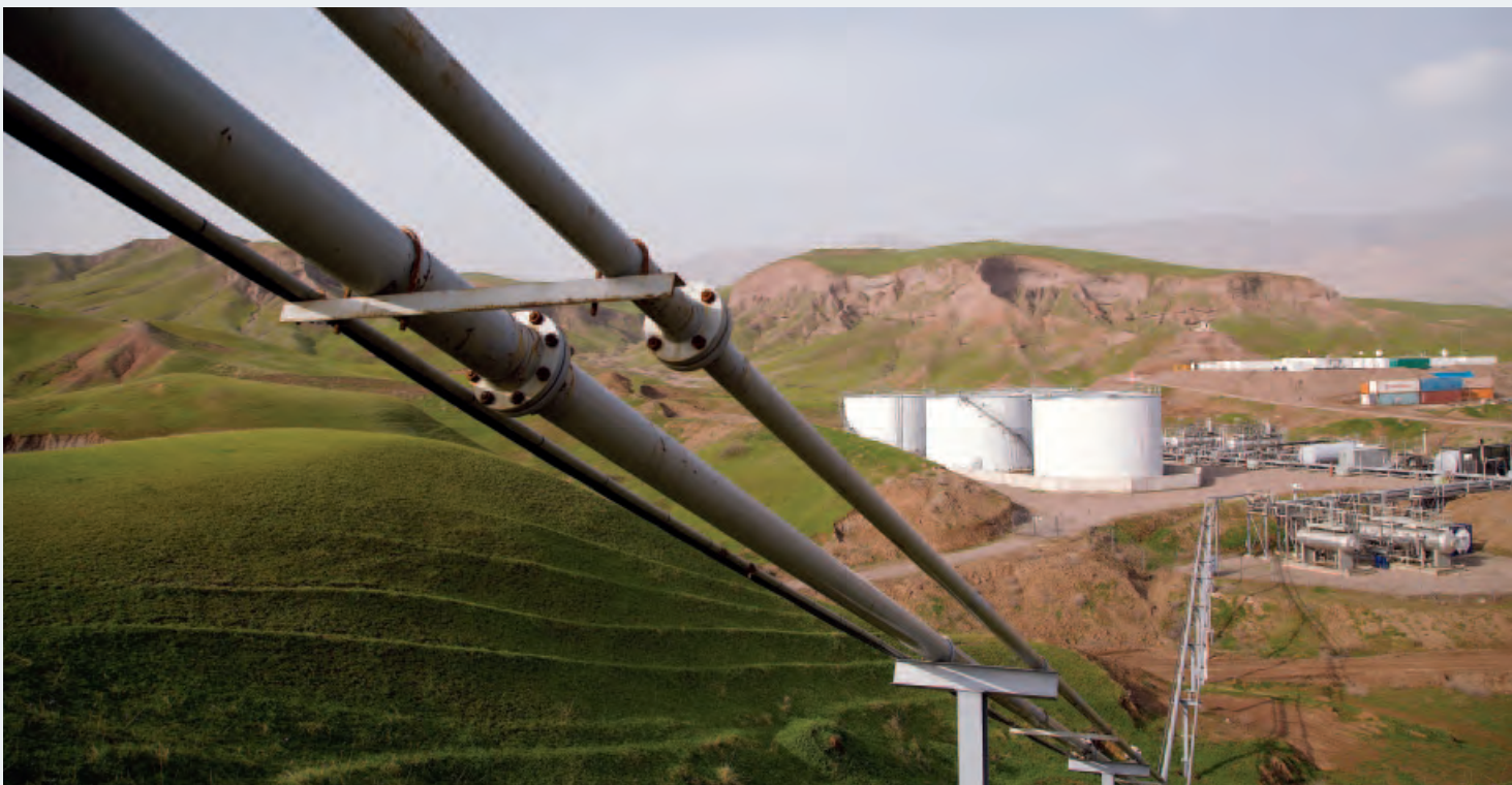
Bijell Early well test facility (EWT)
