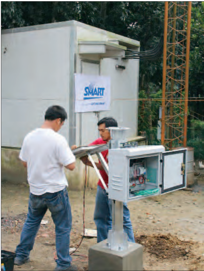
Smart continues to install multiple rain gauges in various Smart cell sites in the country for proper rainfall monitoring.
