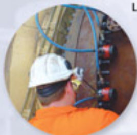
Technical Bolting Services Tensioning, Torquing
