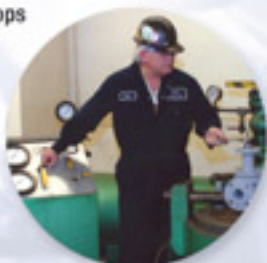
Valve Repair Services Onsite, Inline
