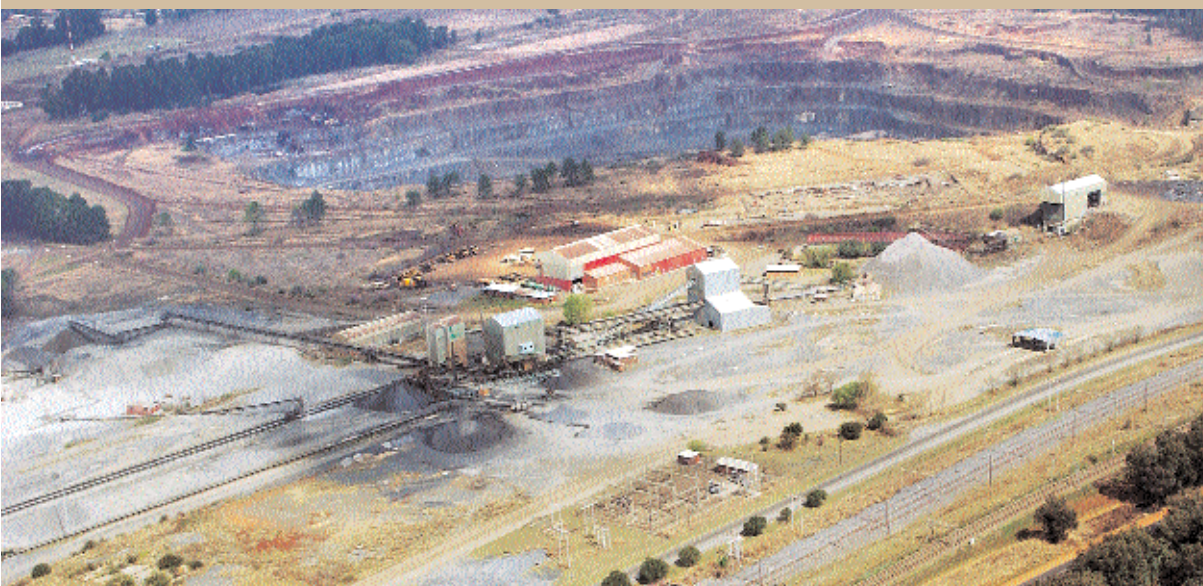
GLEN DOUGLAS MINE
