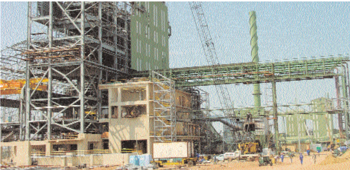
HEAVY MINERALS SMELTER – UNDER CONSTRUCTION
