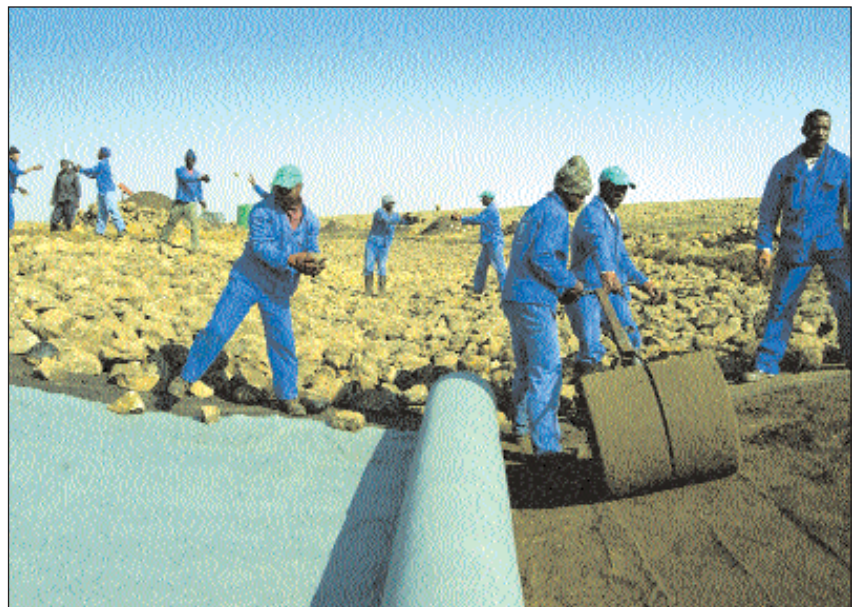
A team sealing the cracks on Hlobane mountain as part of Kumba's pioneering rehabilitation work near the now-closed Hlobane colliery.
