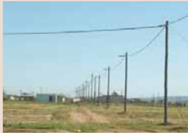
Newly constructed power lines
