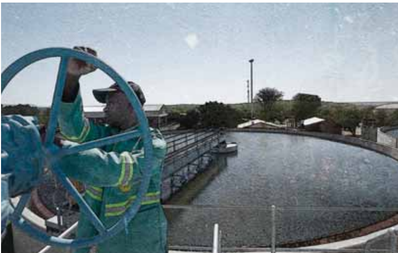
Exxaro's long-term view on water issues means that proactive measures are being taken to mitigate anticipated impacts from climate change
