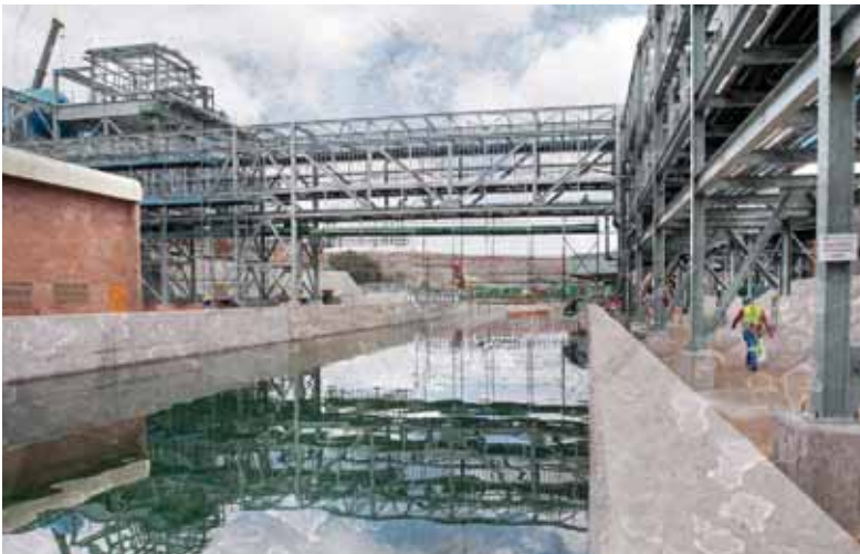
Grootegeluk adopted an integrated water management plan to utilise all surface rain water on the mine premises
