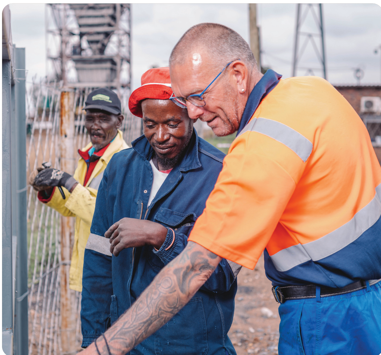
Exxaro maintenance team at work
