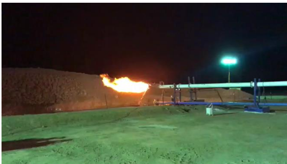
Figure 7 - Albany 1 flow test across a 13 metre interval in the Lake Galilee Sandstone Reservoir.
