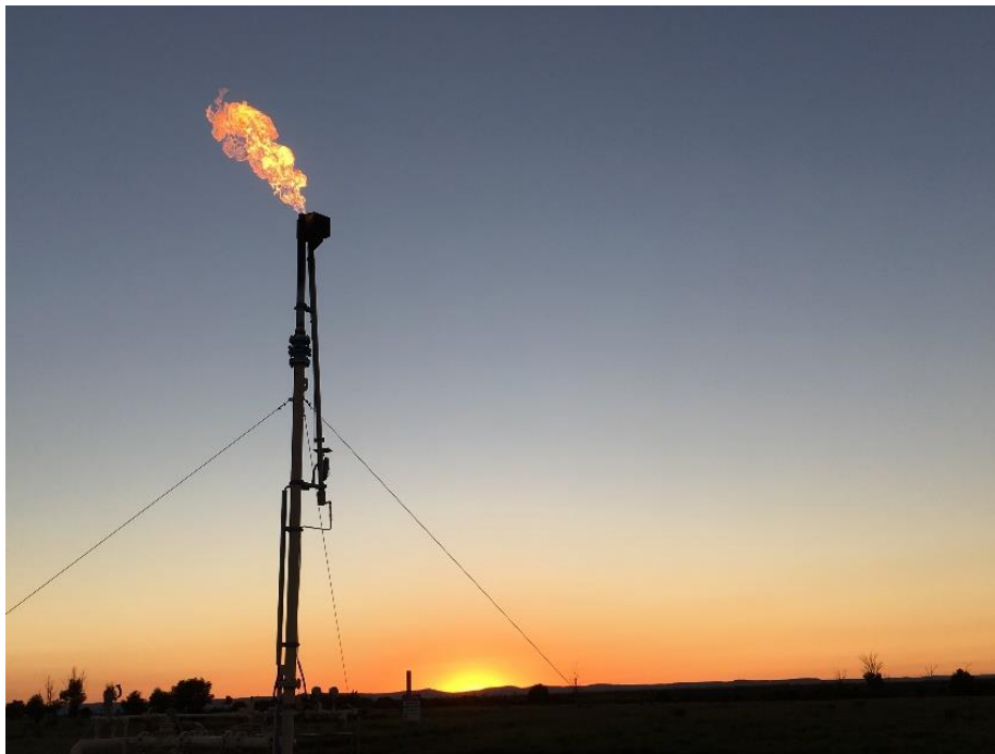
Figure 6 – Flare at Mira Pilot Scheme, Mahalo Gas Project
