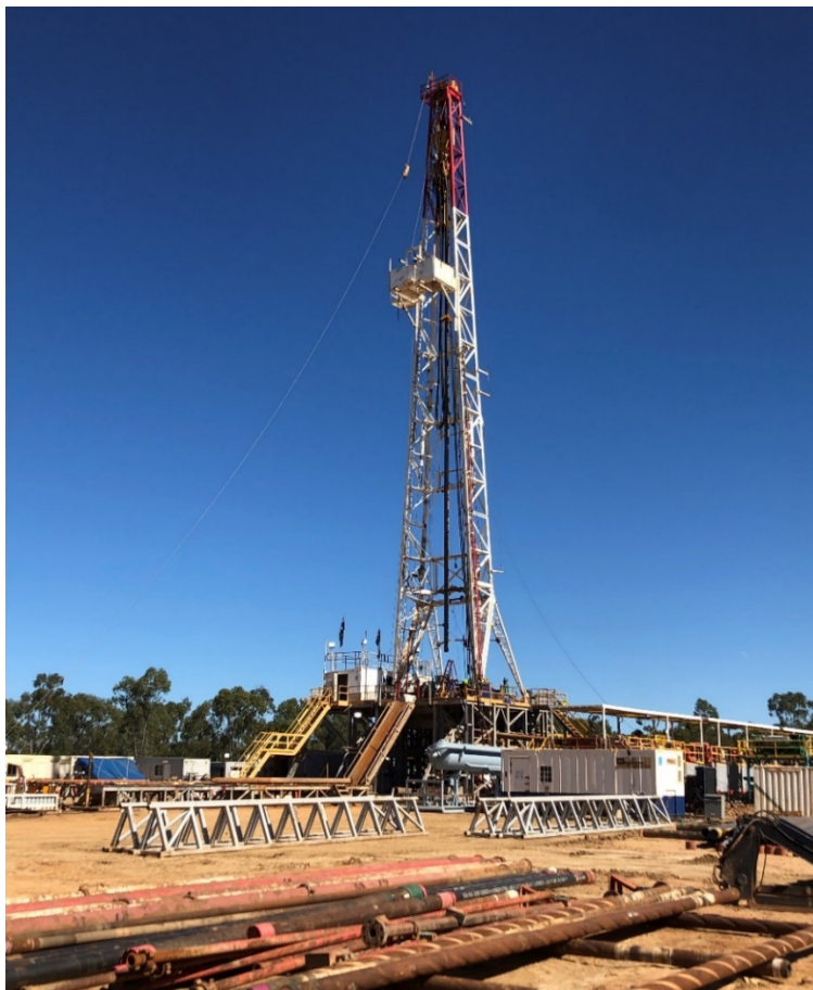
Figure 7 – Photo of Ensign Drilling Rig 932 located at Albany 2
