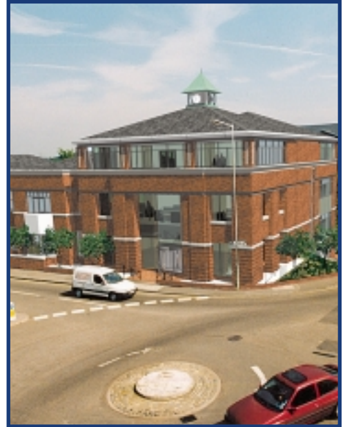
Office development at No 1 Farnham Road, Guildford
