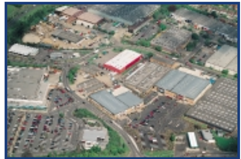
Retail development at Sixfields Retail Park, Northampton
