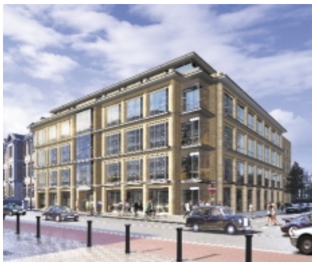
Office development at 200 Hammersmith Road, London W6
