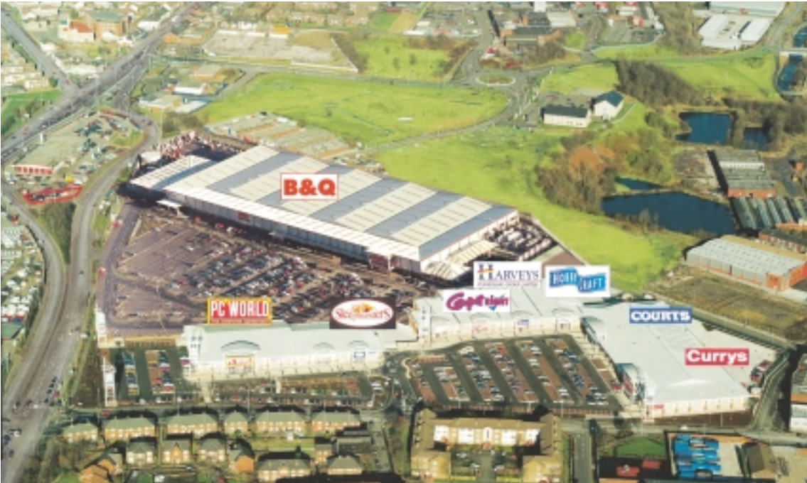
Retail development at Bolton Gate Retail Park, Bolton
