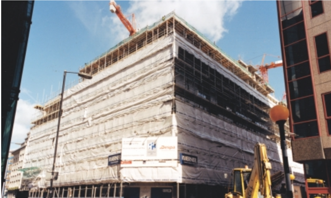
Office development at 25 Chiswell Street, London EC1
