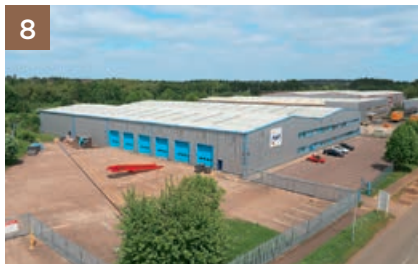
8 CROW LANE, NORTHAMPTON Industrial/logistics
