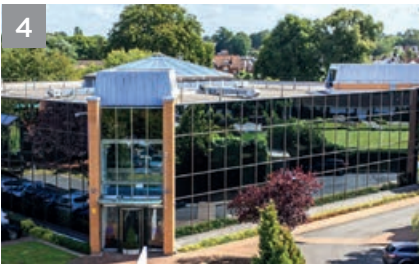
4 THE GLASHAUS, COBHAM Offices
