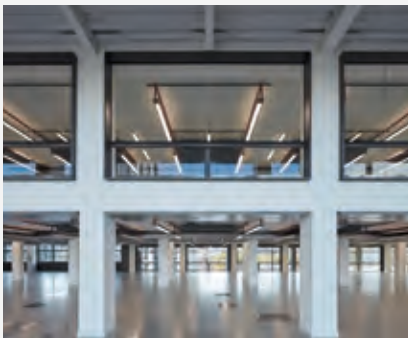
AUG 2018 Phase 2 achieves practical completion
