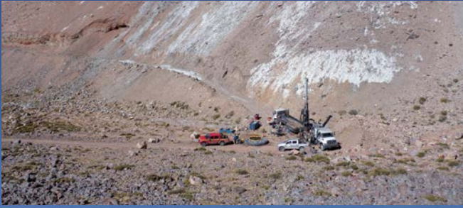
Emplacing water monitoring wells
