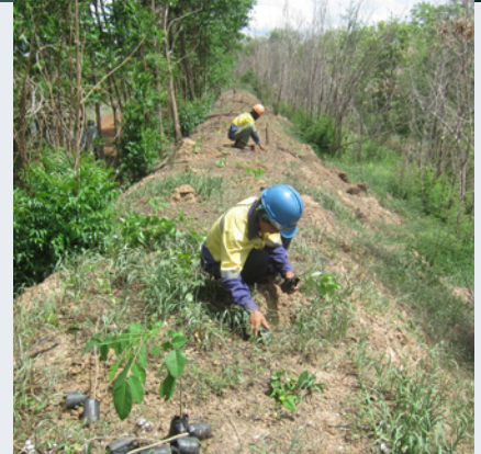
Chatree Environment Department officers managing site rehabilitation: lawn mowing, water sample collection in accordance with DPIM regulations, and tree planting along the ridge of Tailings Storage Facility #2.
