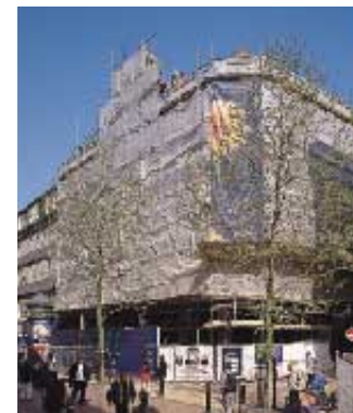
Caxtongate Phase II, Birmingham
