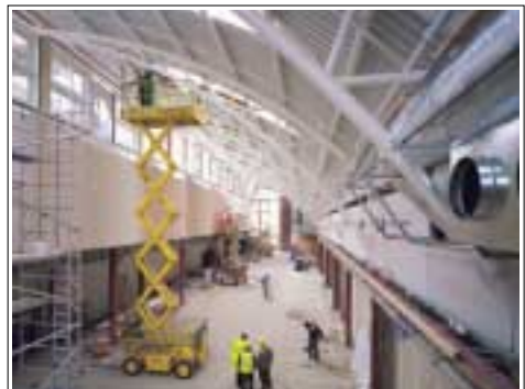
Sunderland – The Bridges Phase II
