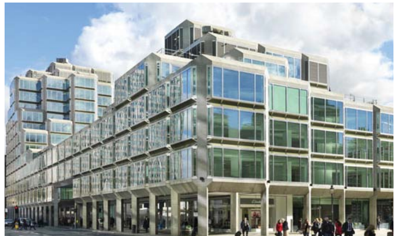
Practical completion achieved at 123 Victoria Street, SW1
